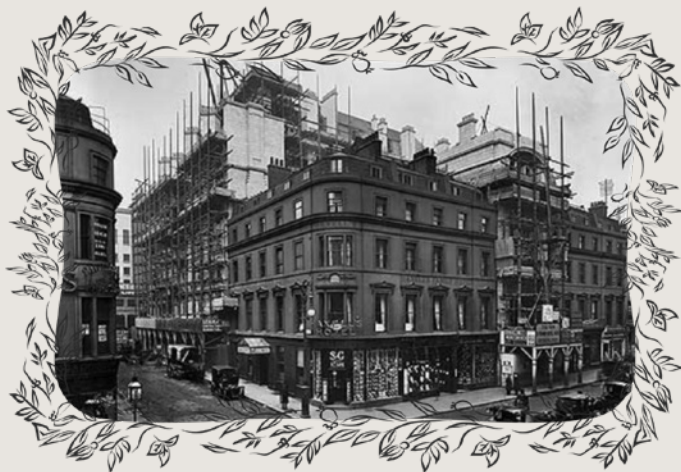
Construction of the Strand Palace Hotel c. 1920s
